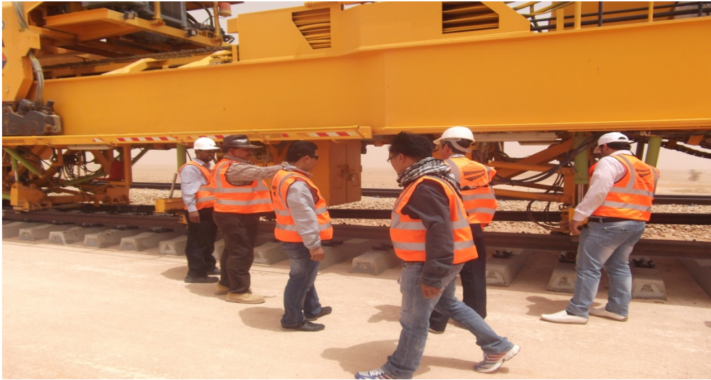
Laying Out Tracks
