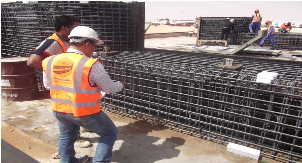
Reinforcement Inspection of Pre Cast Railway Culvert
