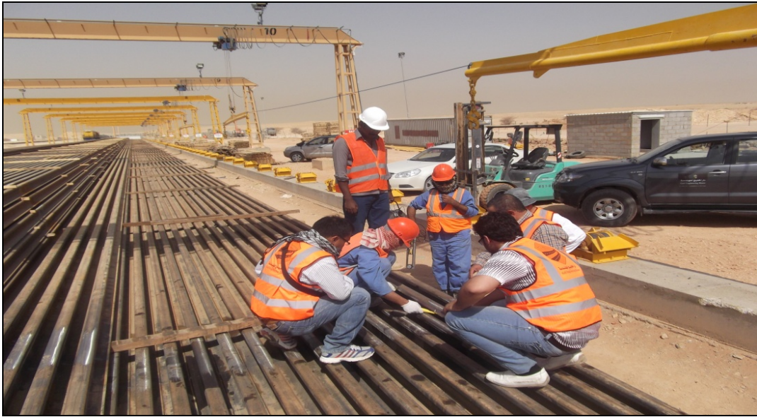
Checking Flash Butt Welded Rails at Fabrication Shop
